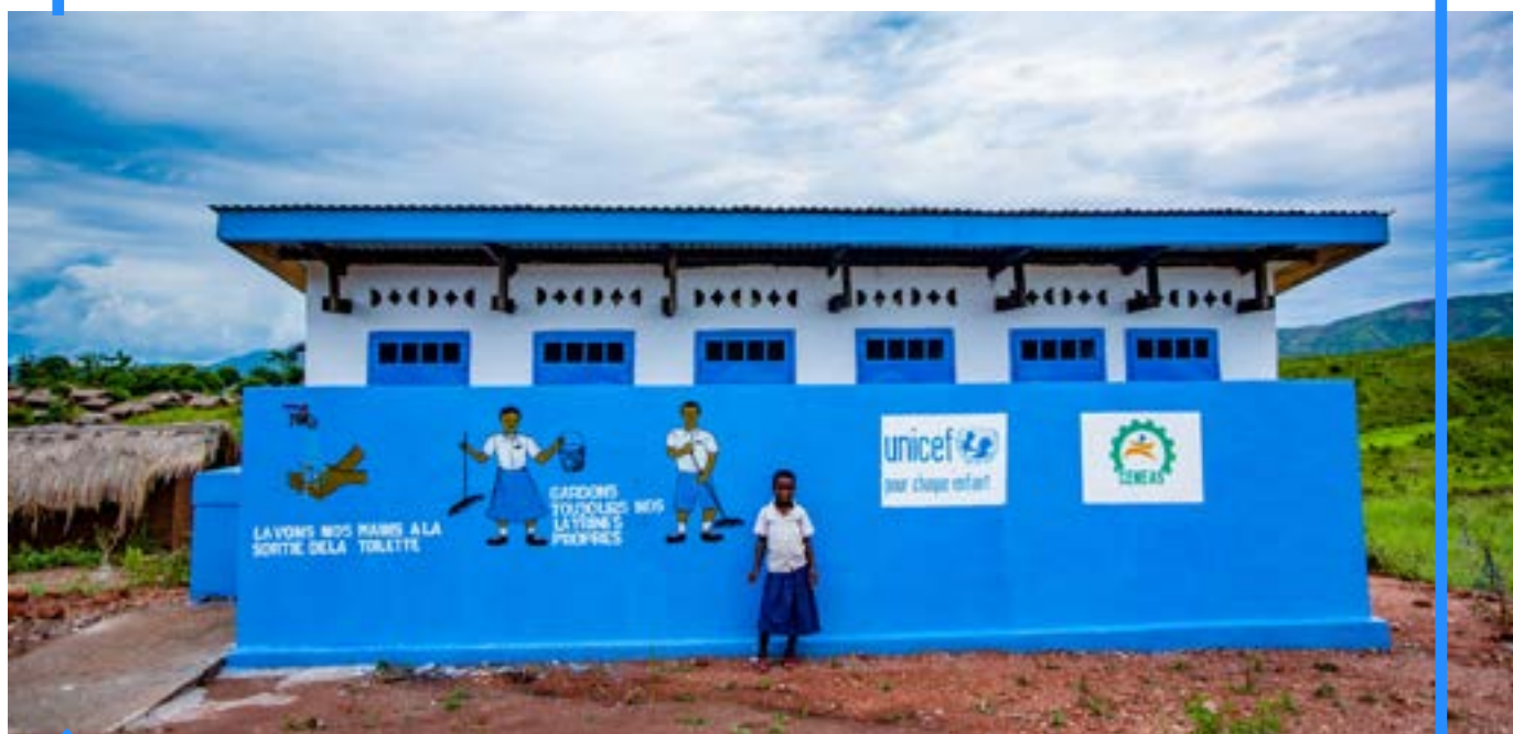
A student stands in front of new latrines at their school in the Democratic Republic of the Congo. The construction of the latrines and new classrooms was made possible by ECW investments.
