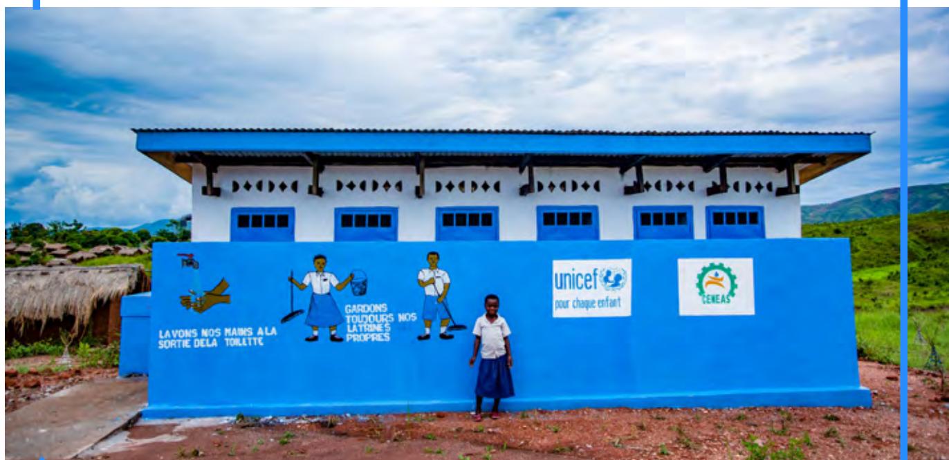
A student stands in front of new latrines at their school in the Democratic Republic of the Congo. The construction of the latrines and new classrooms was made possible by ECW investments.
